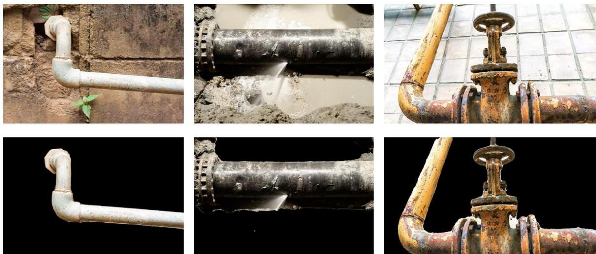
Figure 15: Pipes semantic segmentation results with X-Decoder open-vocabulary: pipe. Source: [63] (left); [64] (centre); [64](right).
