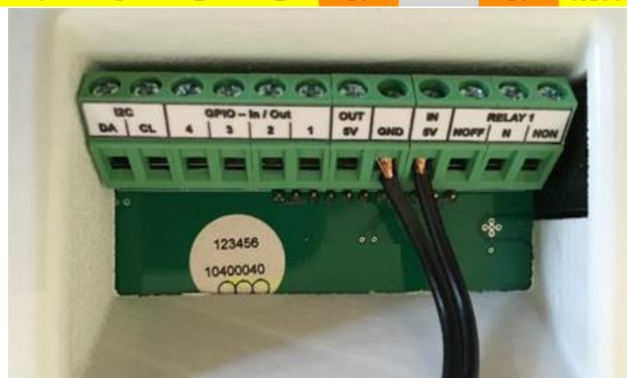
Figure 4: Wiring the terminal block on the back of the terminal
