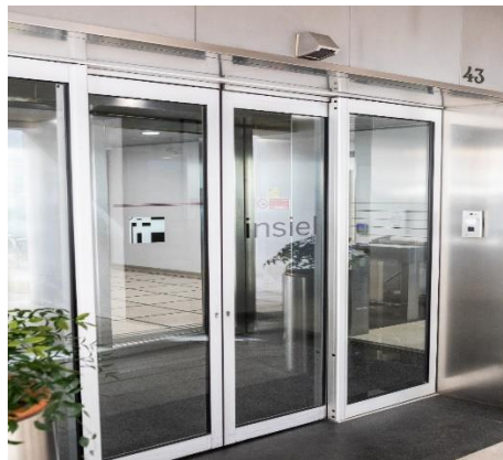
Figure 48: Insiel HQ entrance
