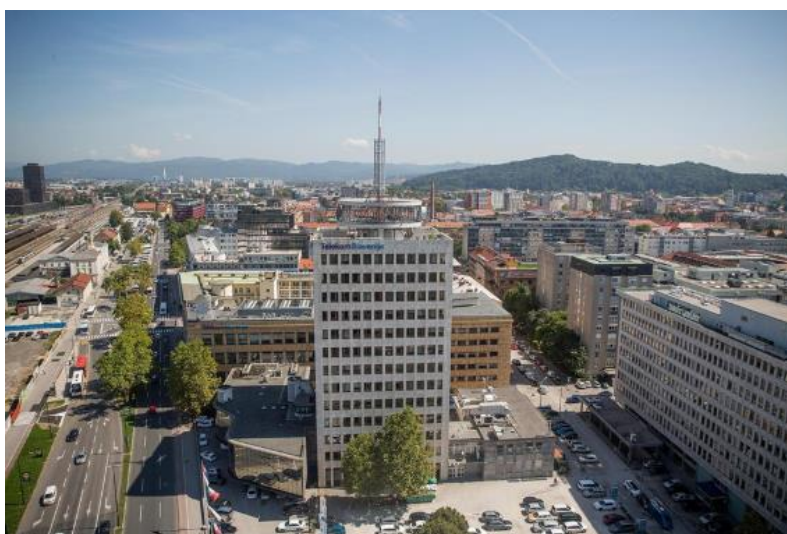
Figure 53: TS offices in Cigaletova street
